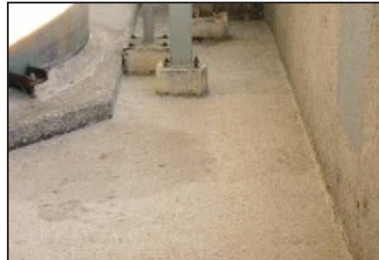
Cleaned and prepared surface
