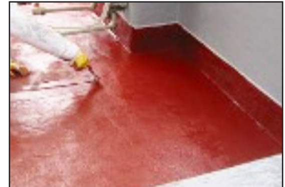
Applying ARC CS4 topcoat
